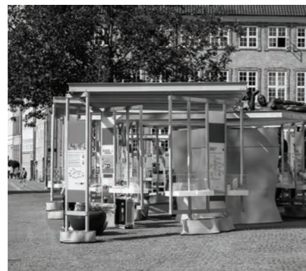
Picture: 5.f Plastic Pavilion Terroir
